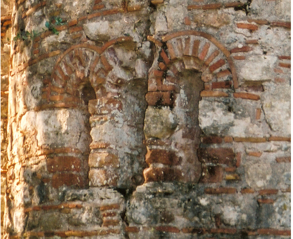
Fig. 46. Stamna, Dyo Ekklesies. Detail of the E façade.
